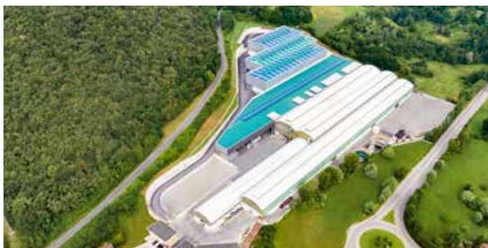
RAFFMETAL Via Brescia, Odolo (BS) RAFFMETAL Street Brescia, Odolo (BS)
